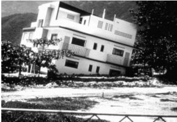
Figure 1. Liquefaction-induced damage following an earthquake in Caracas.
